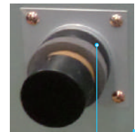
Header pipe sealing
