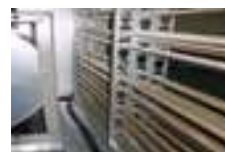
Electric heater section
