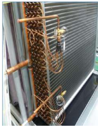
Figure 4: Water & DX System Coil
